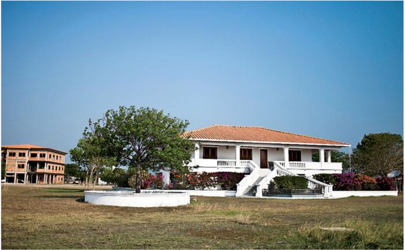
Photo: The Unification Settlement Puerto Leda
